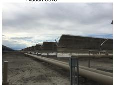
Concentrating Solar Assist for Geothermal Plant
